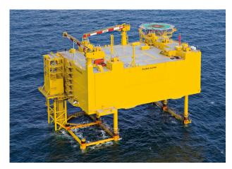
Self-installation allows platform components that would exceed the capacity of the largest barges to be assembled cost-effectively.
